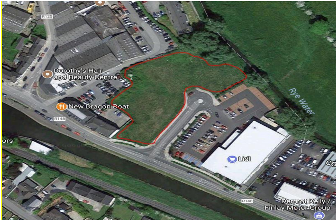
FIGURE 1.1 Site location adjacent to Lidl and north of R148
